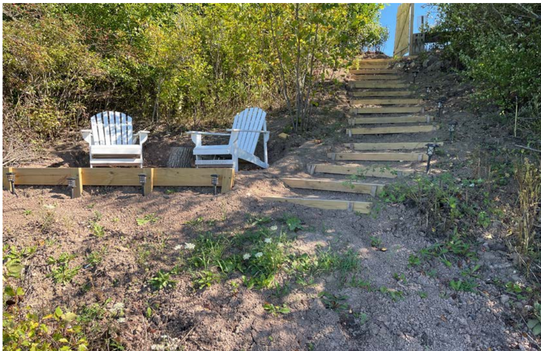
Photo 8 - Note exposed clay along slope at Site No. 91.
