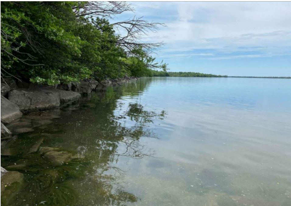
Figure 4. Photo of rip rap along shoreline, Site 91
